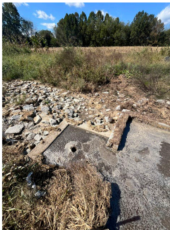
Chunks of silage and leachate which has overflowed from the catch basin. The catch basin is clearly clogged, which allows a discharge over the sides and into a rock channel which leads to the wetlands which leads to Basin Run.
