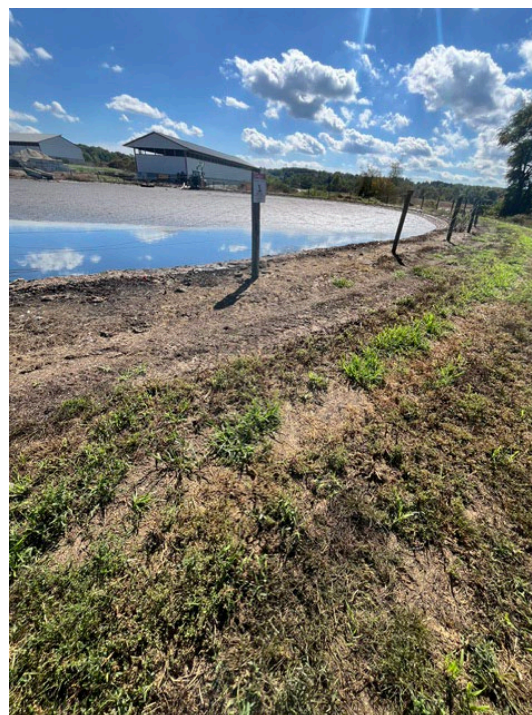
Manure pit #3 west side showing evidence of a previous overflow.
