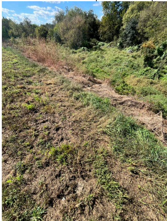
Dead or dying plant life showing the probable path that a manure overflow took from manure pit #3
