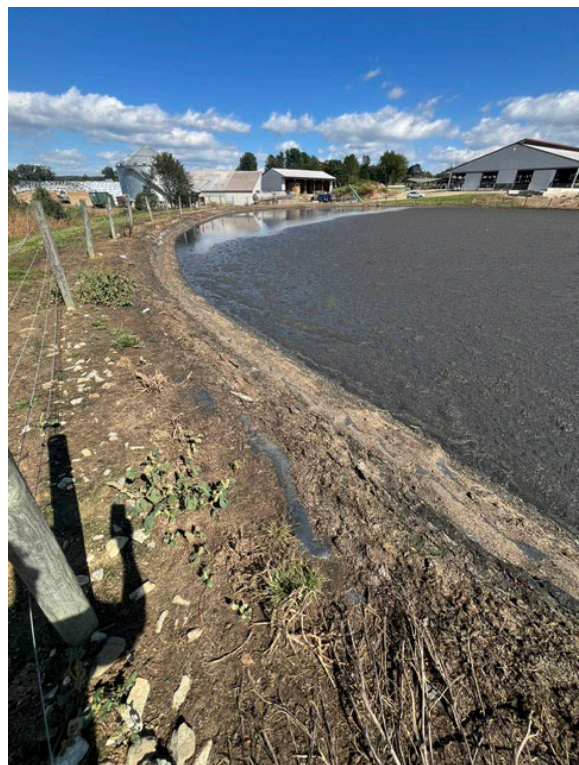
Manure pit # 3 shows evidence of a recent overflow
